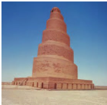
Minaret from the mosque at Samara
